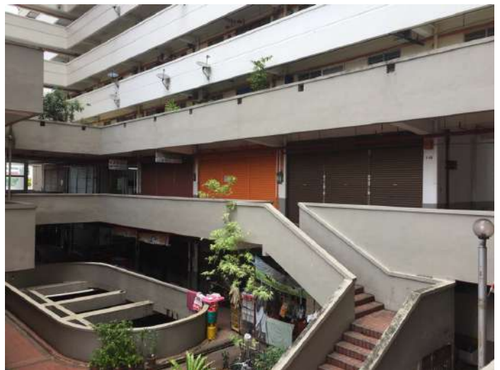
Figure 11: Ground floor, Jalan Kedah Flats. (Source: Think City)
