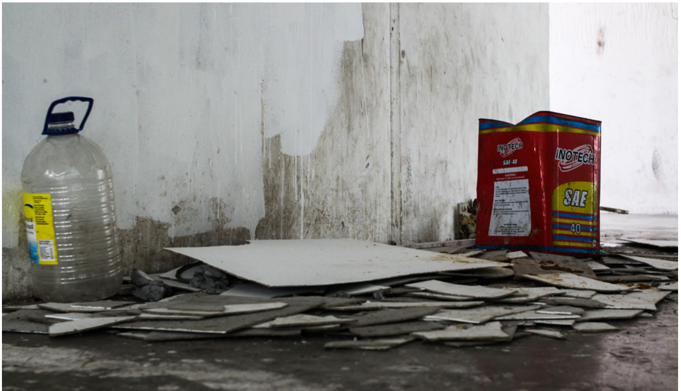
Figure 14 Rubbish dumping in stairwell — a health, safety and liveability issue Source: Think City
